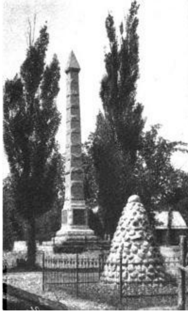
Figure 8: Two monuments to the victims of the Spirit Lake Massacre. In the foreground is a cairn of stones that settlers and visitors to the site erected, apparently spontaneously, as a show of respect for the dead; behind it is the obelisk erected by the State of Iowa in 1895. The roof of the Gardner family cabin can be seen in the right background. Placement of the new monument next to the old one signals the direct link between the frontier past and the modern present. Agnes C. Laut, "Pioneer Women of the West: The Heroines of Spirit Lake, Iowa," The Outing Magazine , LI (October 1907-March 1908), 693.
